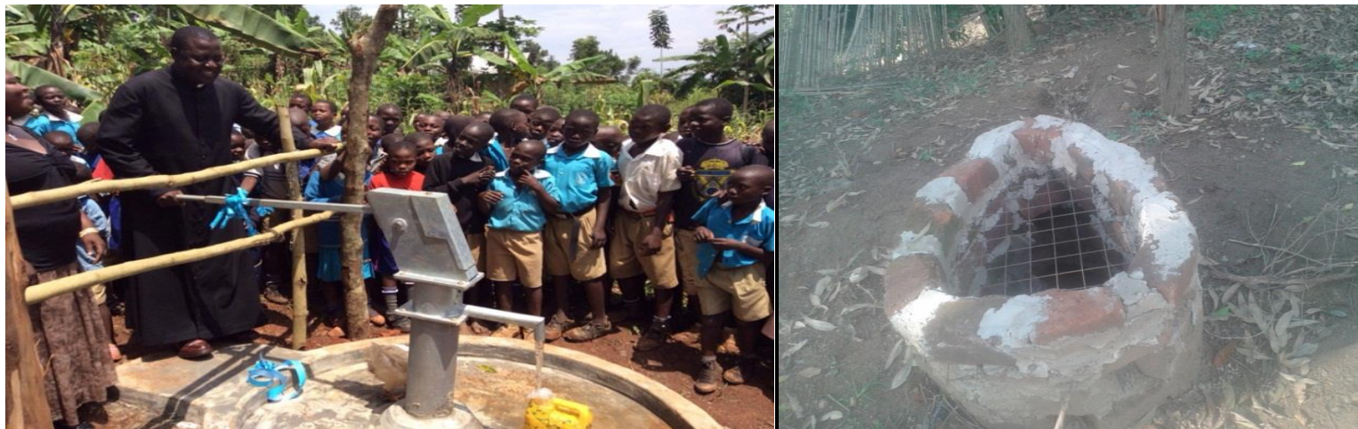
Fr. Paul Ssebitoogo launching the newly constructed borehole for Kasenge R/C p/s by the church and an incinerator at Sekiboobo p/s respectively.
